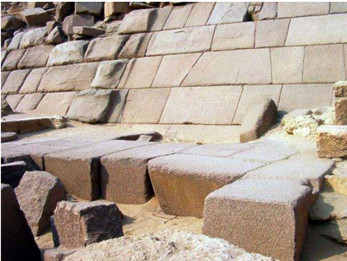
Figure 16. A view of the unfinished granite casing and floor of the Menkaure Pyramid, where the sample for OSL dating was taken. Note how only the central portion of the casing of each Pyramid's face was smoothed, whereas the remaining blocks were left in the rough. Image in the public domain. From Wikipedia.
